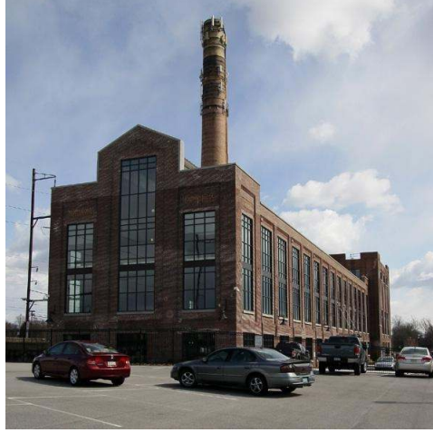
Fig. 5: Tarihte Ambler Boiler House (Philadelphia).
