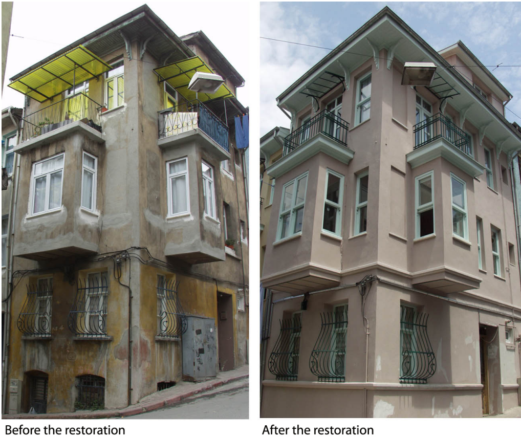
Photo 3. Fener Balat Rehabilitation Project (URL-4, 2011)
