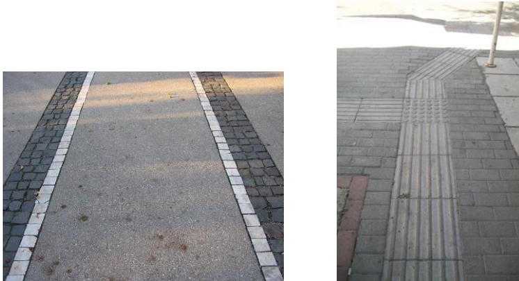
Figure 1. Tactile guiding lines/strips
