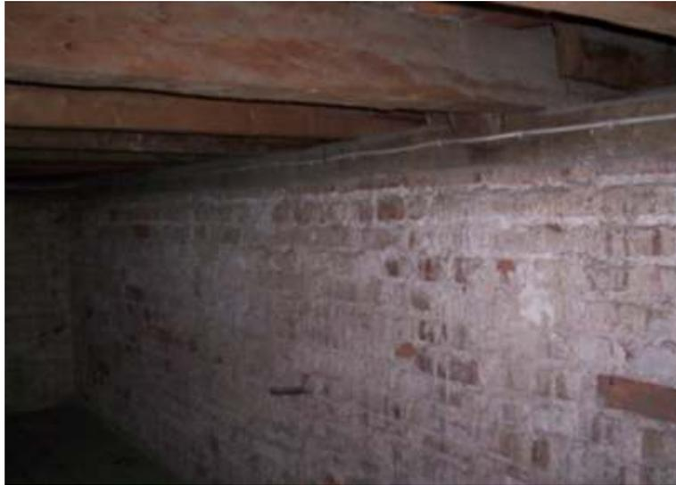
Figure 3. Structural wall and timber slab in the roof of the structure.
