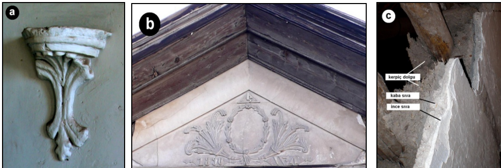
Figure 6. [a] Gypsum lamp stand, [b] Gypsum decoration on façade of structure B and its date of construction, [c] Plaster layers.
