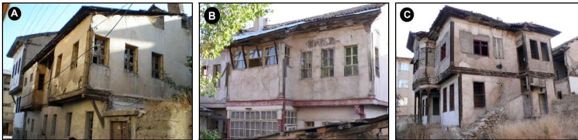
Figure 1. [a,b,c] Various structure samples in Sivas whose internal and external facades are plastered with sweet plaster.
