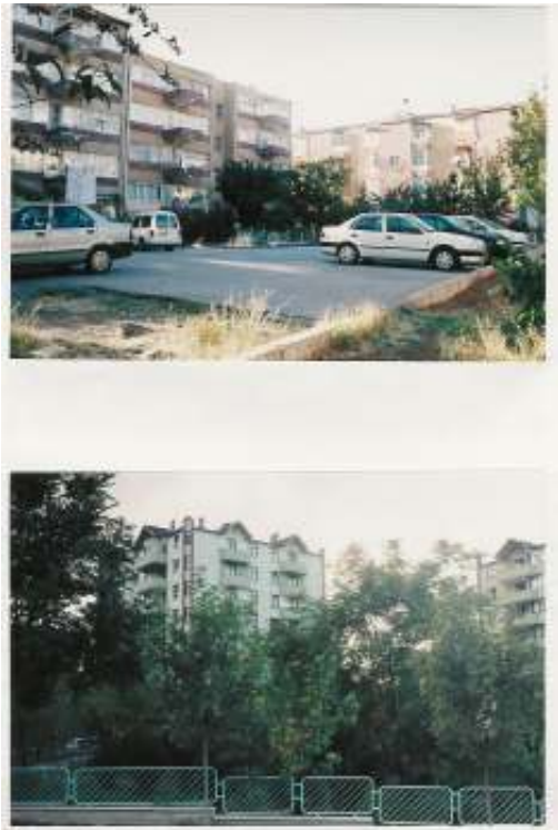
Figure 6: Fenced residential blocks
