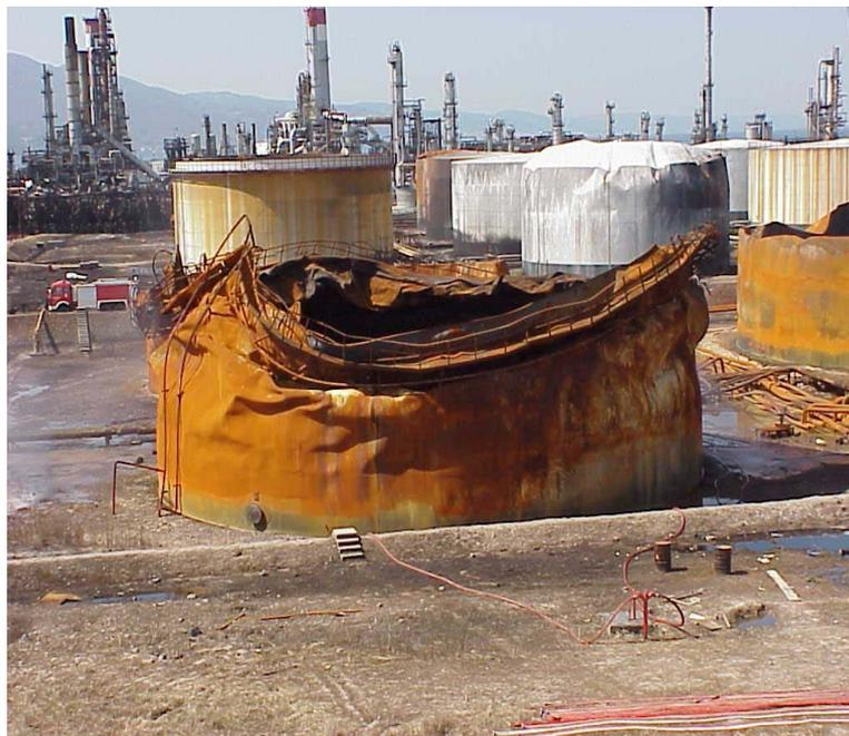
Figure 1. Naptha fuel storage tanks damaged by fire resulting from the earthquake at the Tüpraş Refinery, Izmit the structure–liquid and structure–ground interactions [7].
