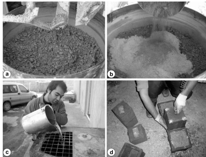
Figure 6: Preparation of concrete mixture (a-d).
