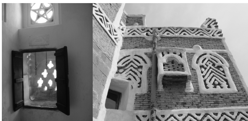
Figure 1. Interior view of a cold weather storage window (left) and exterior view of another cold weather storage window (right) in the House of Imam Yahya, Sana, Yemen [16]
