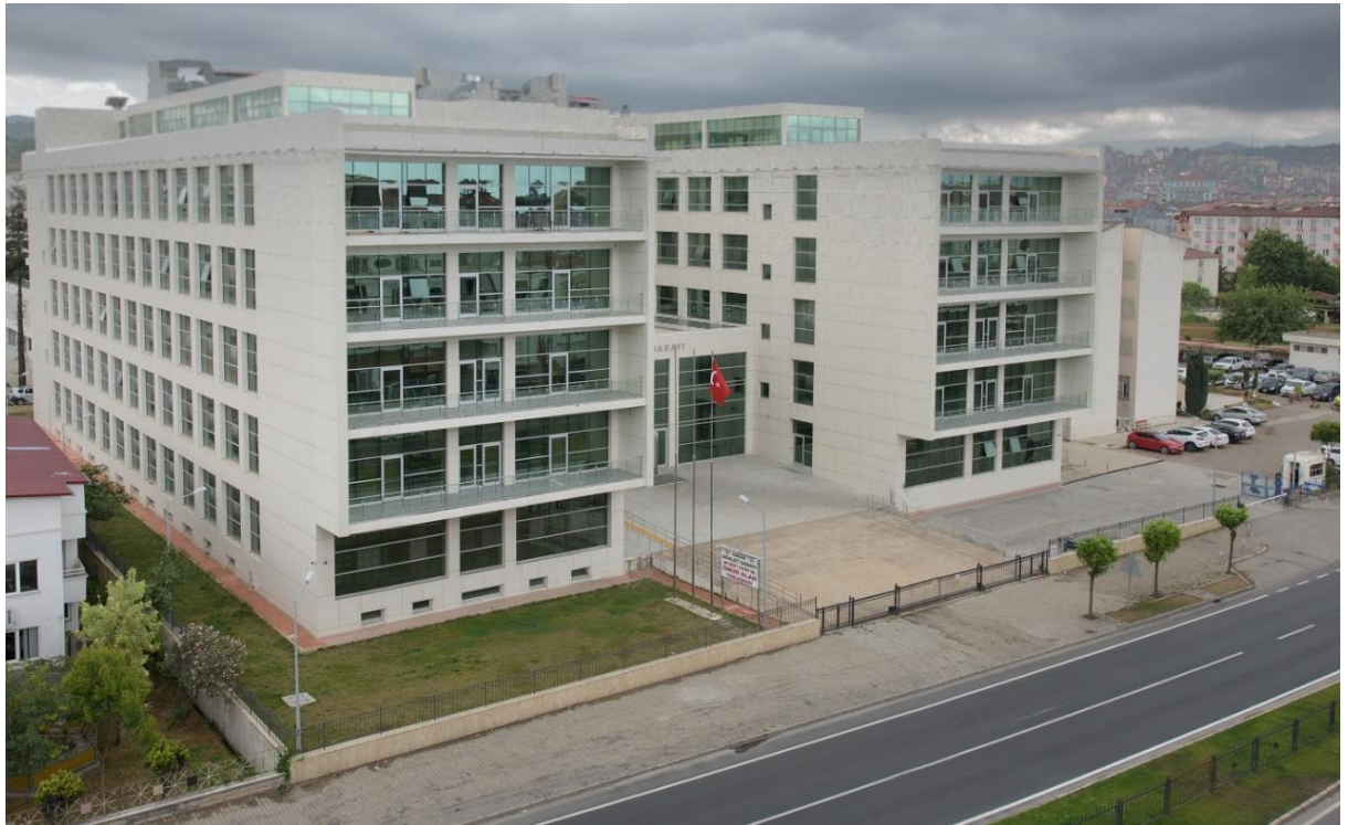
Figure 10: Exterior view of Ordu Annex Courthouse Building
