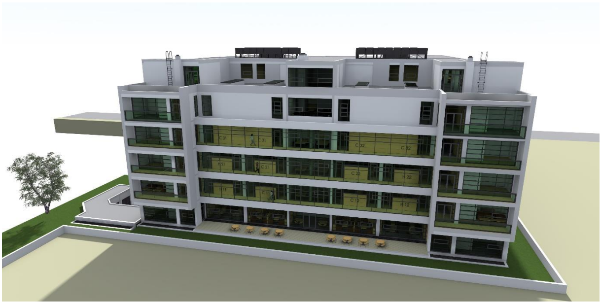
Figure 5: South Facade of the Building - Judge Corridors are Showed
