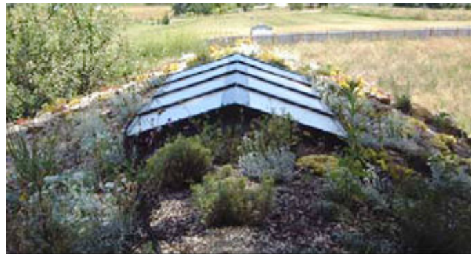
Figure 3. Green roofs and solar panels
