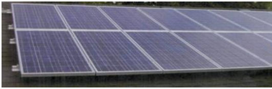
Fig 1. A typical PV Array Individual modules are attached to a racked system and wired together to form an array [10].
