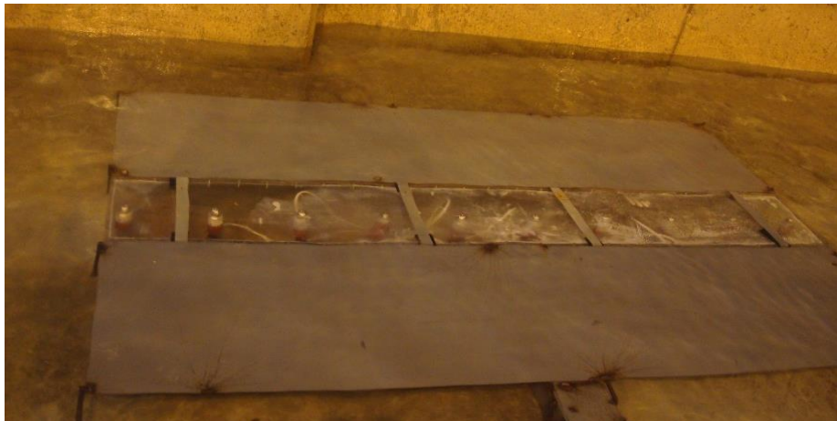
Figure 2. Installment of Pressure transmitters on the channel floor
