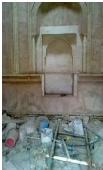
Figure 5: A view of the interior monuments, before restoration
