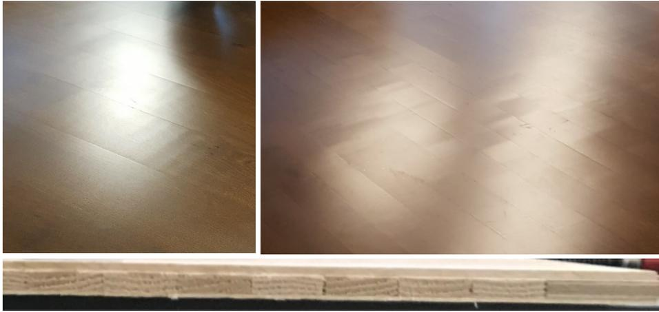
Figure 1: Above: Ondulation at finished multi-layered (laminated) parquet surfaces
