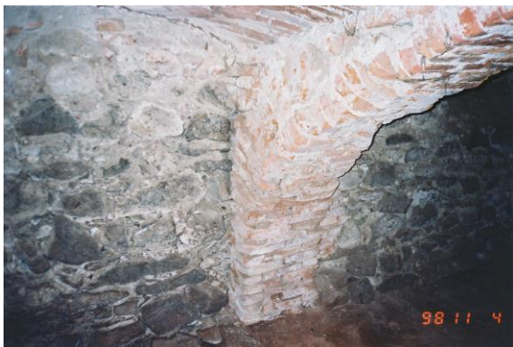
Fig. 3. Masonry stone walls, brick arch and vault
