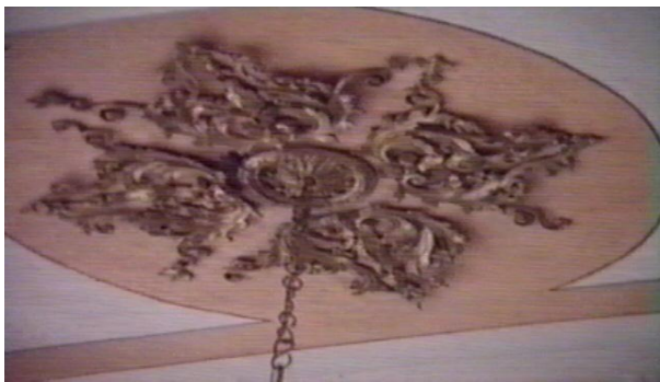
Fig. 5. Plastering in stucco of the ceiling
