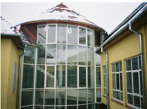
Fig. 11. New staircase - exterior view
