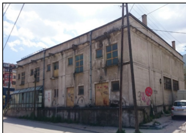
Figure 3. Previous condition of the building (exterior) b
