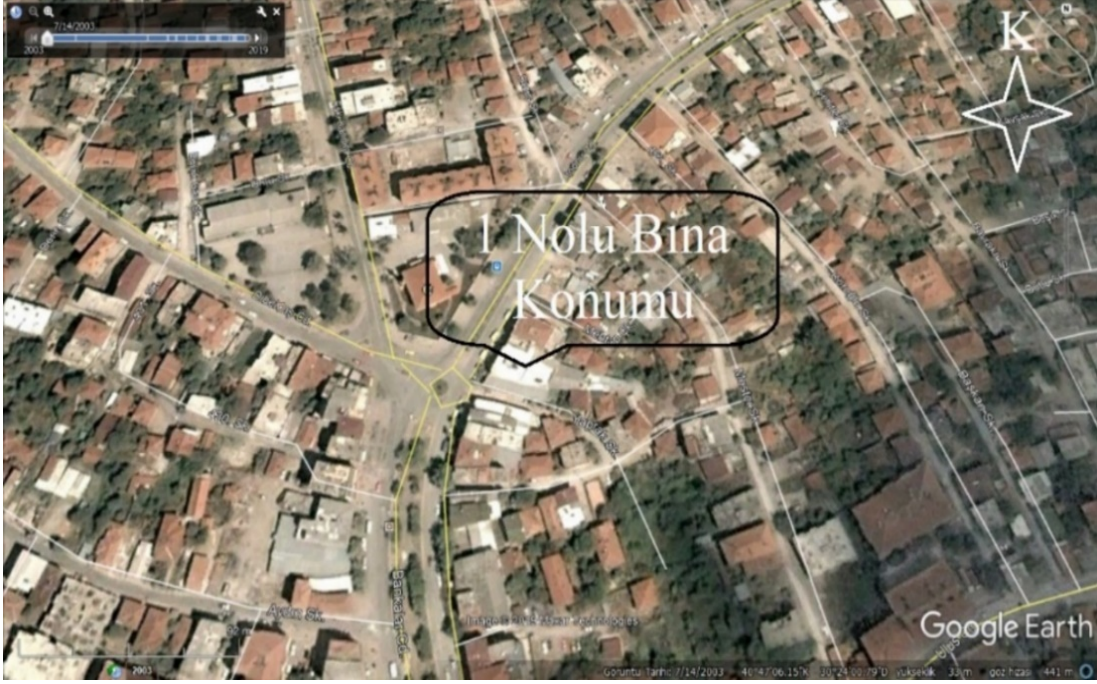
Şekil 4. 1999 Adapazarı Depreminde Devrilen 1 Nolu Binanın Konumu, [2] (Location of Building #1 Which was Overturned in 1999 Adapazarı Earthquake)
