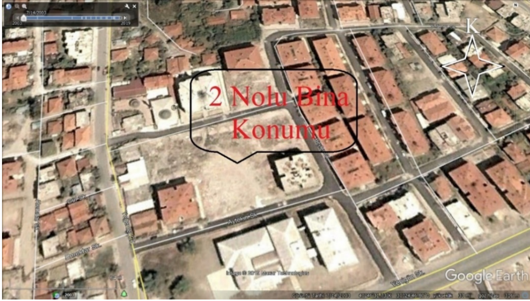
Şekil 6. 1999 Adapazarı Depreminde Devrilen 2 Nolu Binanın Konumu, [2] (Location of Building #2 Which was Overturned in 1999 Adapazarı Earthquake)
