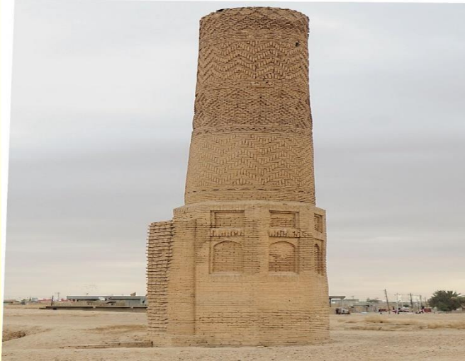
Ek 3 Dakuk Ulu Camii Minaresi ( http://www.selcuklumirasi.com/architecture-detail/dakuk-ulu-camii-minaresi )
