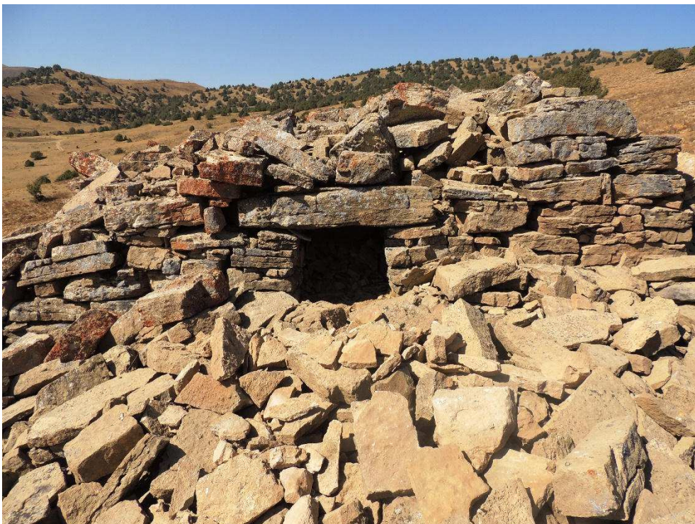
Fig. 42. Construction no 4 with window or entrance
