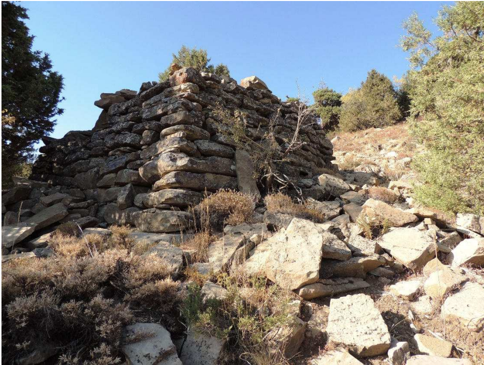
Fig. 35 Construction no 13 east-southern side.
