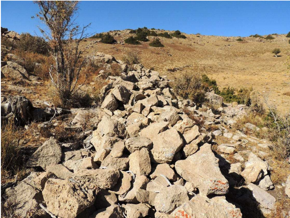
Fig. 19 Wall separating citadel from shahristan. East-west direction.
