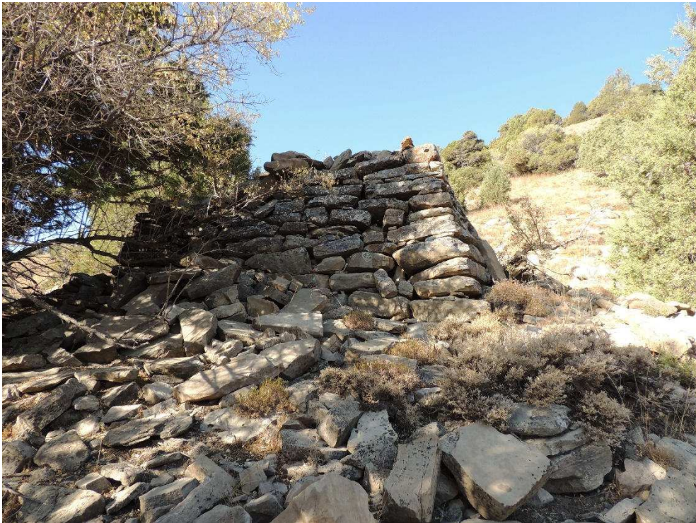
Fig. 34 Construction no 13 eastern side.
