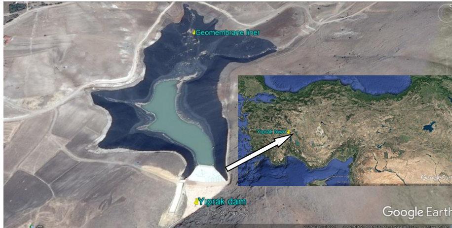
Fig.1. Google earth view showing Yiprak dam (Google Earth view).[9]
