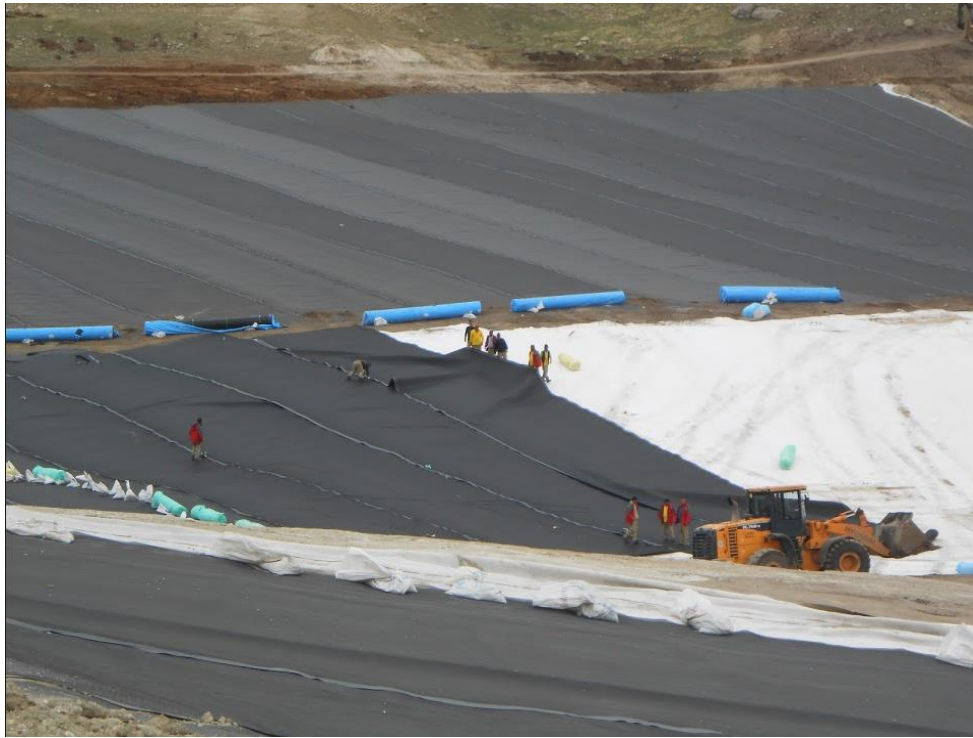
Fig. 3. A view showing reservoir lining for pervious bedrock
