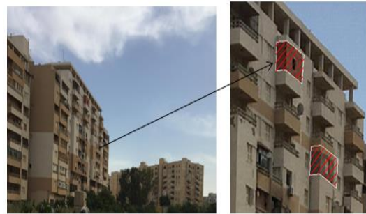
Closed the balconies by users- EL-Hadba Housing project
