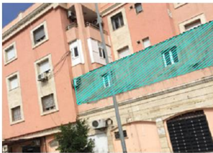
Closed the balconies by users - Ghot Ash - Ahaal Housing project
