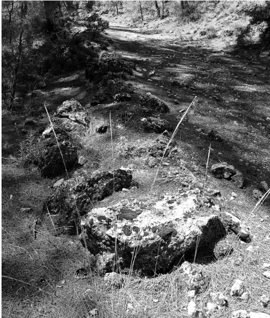
Fig. 14 Remains of some retaining walls of the old road from Bel near Sidyma
