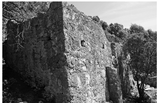
Fig. 39 Gavur Kalesi. Detail of the masonry
