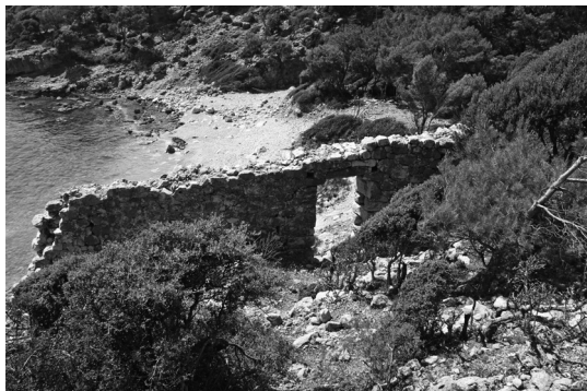
Fig. 35 Gavur Kalesi. Entrance to the west
