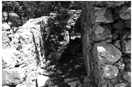
Fig. 40 Gavur Kalesi. Detail of the passages
