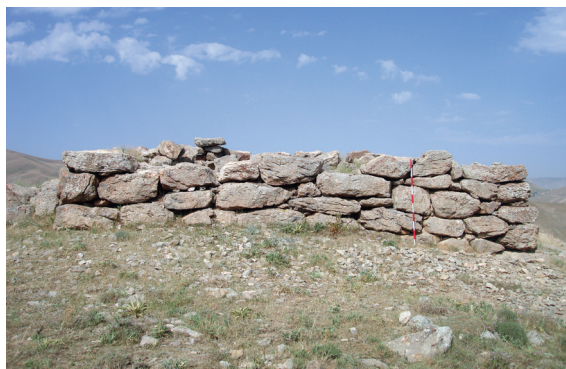
Figure 5- View of the Malkofri structure from the East.
