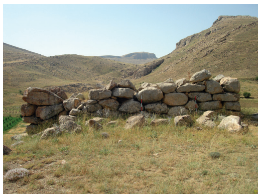
Figure 8- View of the Zerrin Dol-1 structure from the north.
