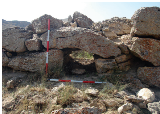
Figure 6- View of the opening in the north wall of the Malkofri structure.
