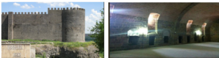
Photo 3a, 3b: Diyarbakır Castel, Diyarbakır, TURKEY
