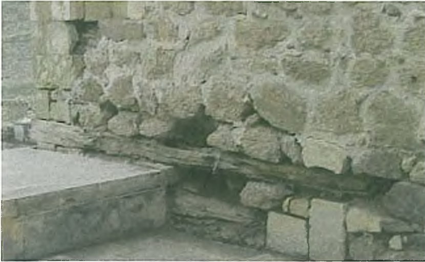
Figure 2. Wooden beams of Ishak Pasha Palace. (Erdoğan, 2006)
