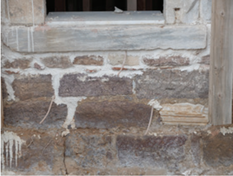
Figure 17. Detail of Tuzla Hüdevendigâr Mosque east façade window (2019)
