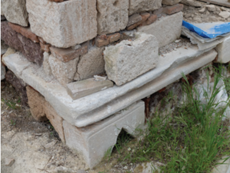
Figure 25. Detail of Tuzla Hüdevendigar Mosque narthex(2019)
