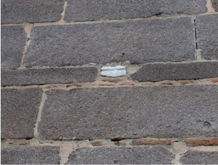
Figure 5. Detail of Behramkale Hüdavendigâr Mosque western façade (2019)
