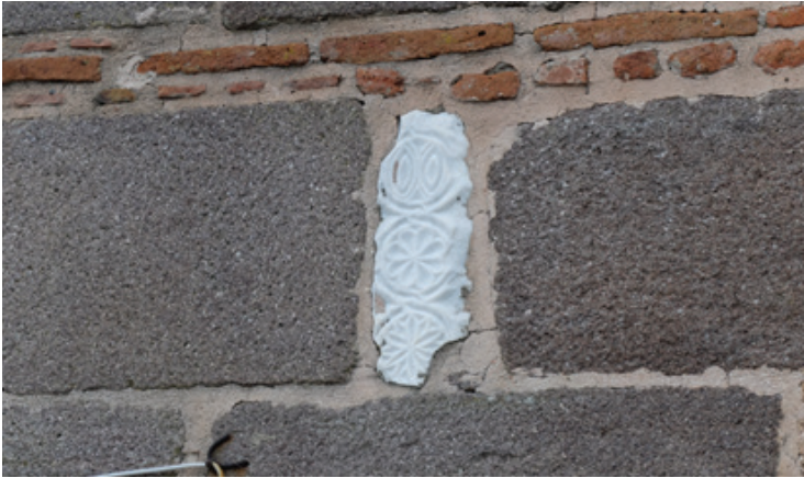
Figure 6. Detail of Behramkale Hüdavendigâr Mosque western façade (2019)
