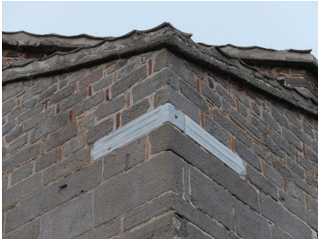
Figure 2. Detail of Behramkale Hüdevendigar Mosque south east corner (2019)
