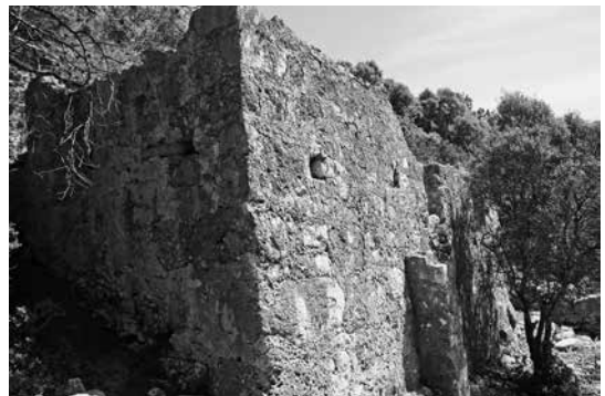
Fig. 39 Gavur Kalesi. Detail of the masonry
