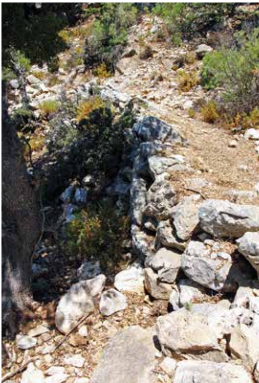
Fig. 47 Road descending in the direction of bay of Gavur Kalesi
