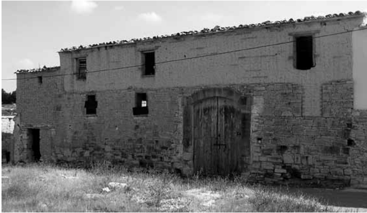
Fig. 11 Khan, Building A, south elevation towards street; left: unassociated passageway
