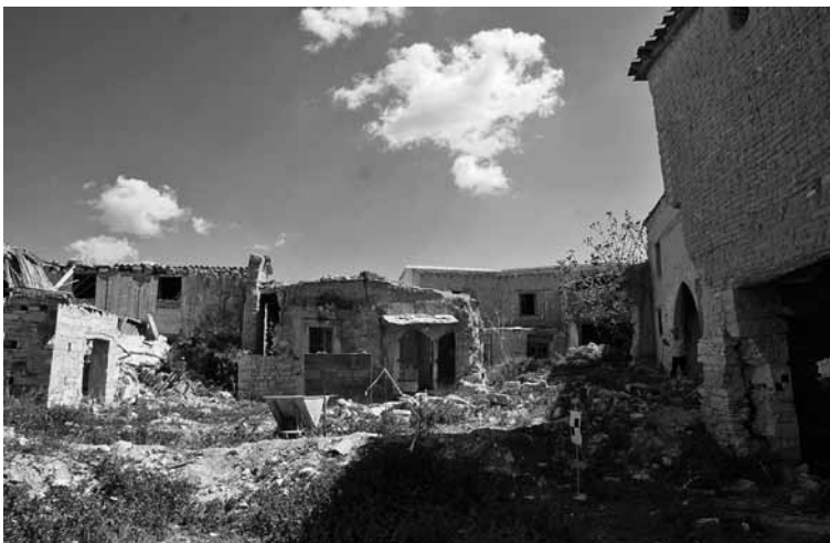
Fig. 8 Khan, view towards east over destroyed Building B and trench markers onto unrestored facades of Stable E (left in front), Guesthouse F, Coffee house G (center), H (right), A (far right) and unassociated passageway (far right/in front)
