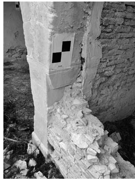
Fig. 15 Khan, Building A, rest of filling of middle arch and ashlar pillar with capital
