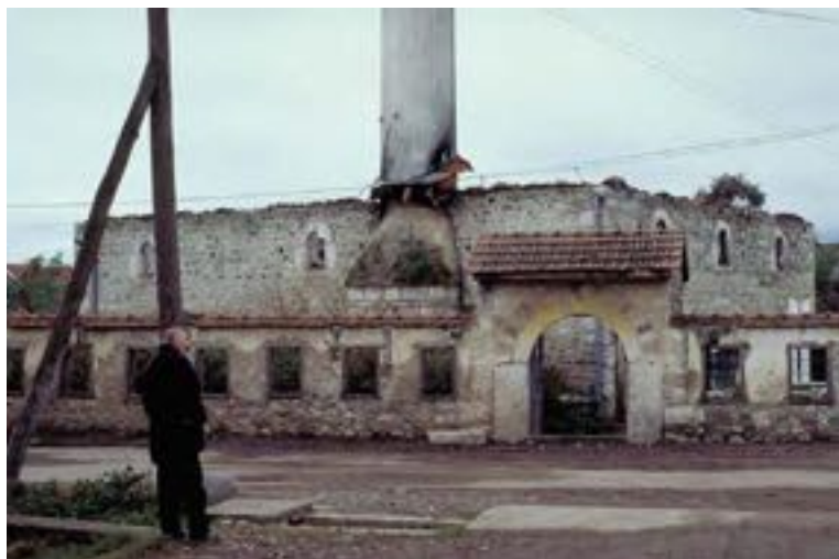
Figure 2. Mosque in Deçan burnt during the '98-99 War (Riedlmayer, 2014)
