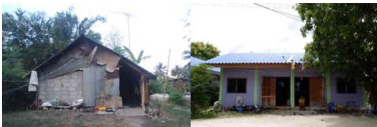
Figure 3. The change of a house of a squatter who joined the project in 2010. In 2012, he demolished the old house (left) built from bricks and galvanized iron sheets, and he built a new twin house (right) for himself and his daughter.
