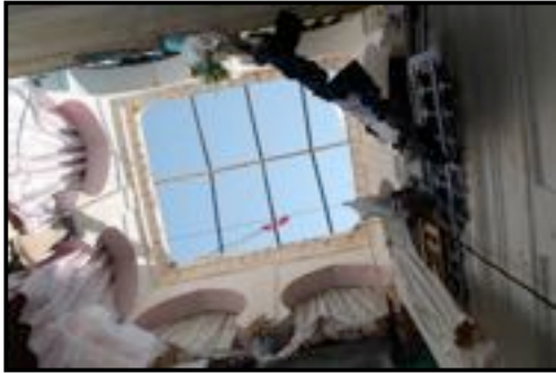
Figure 8. Roof top view, Source: Author
