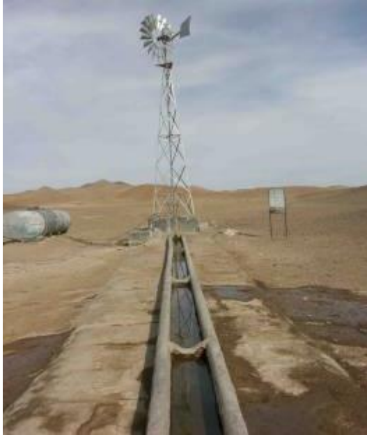
Figure 4. Establishing a wind water pump.
