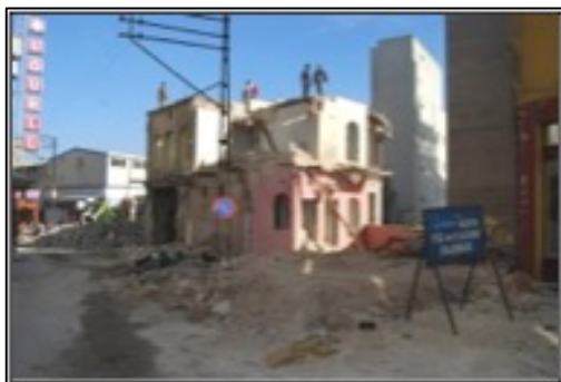
Figure 24: Street Widening Works
