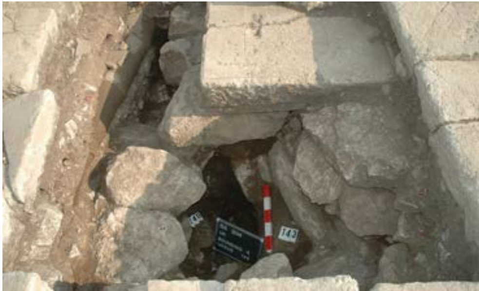
Fig. 2: View of the pit (locus 140) dug into the ophiolitic clay (locus 143), and of the overlying foundations of an honorific monument on the Upper Agora (Sagalassos Project).
