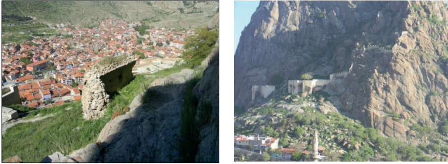
Figure 11: Middle Castle's vaulted building remains and city walls (Köker, 2020)
