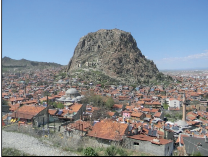
Figure 1: Afyonkarahisar Castle Southeast Facade (Köker, 2020)
