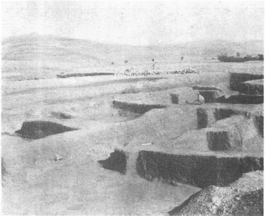
Fig: 2 — View from southeast towards group of rooms forming the north block in the Level I fortress at Hacilar
