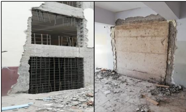
Figure 4. Adding shear walls
