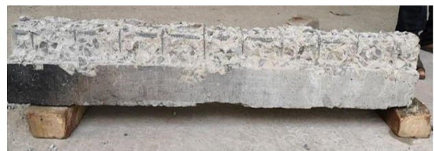
Figure 6. Chiseling of beam
