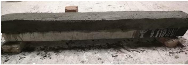
Figure 7. External strengthening of beam
