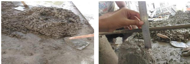
Figure 2. Preparation of Concrete
