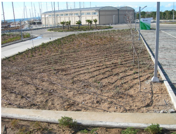
Figure 12. Parking Lot Area, 2009 (Balik, 2021b)
