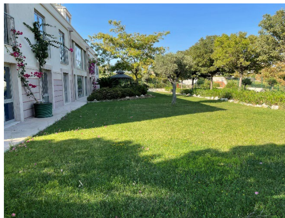
Figure 61. Administration Building: Rear Section No.1, 2021 (Balik, 2021b)
