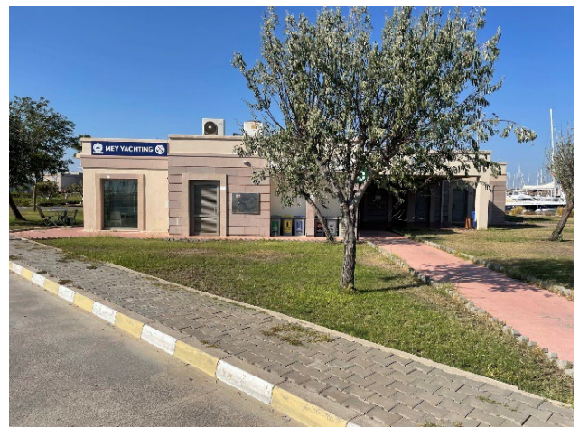
Figure 77. Berth Area: Northeast No.2, 2021 (Balik, 2021b)
