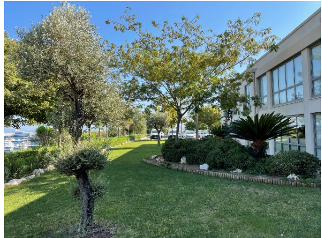
Figure 63. Administration Building: Rear Section No.3, 2021 (Balik, 2021b)
