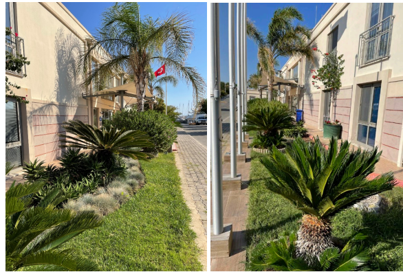
Figure 59. Front Section of the Administration Building, from Left and Right, 2021 (Balik, 2021b)
