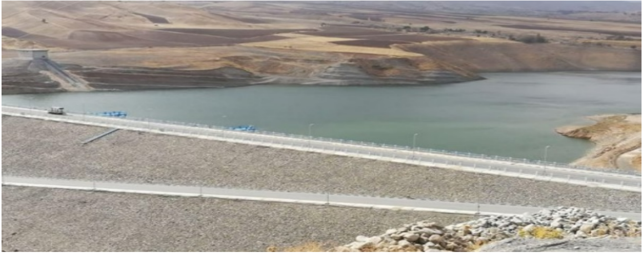
Figure 1. Overview of Silveh Dam.
