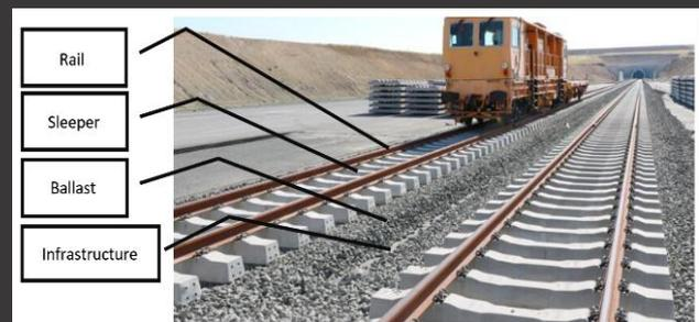
Figure 1. Representation of conventional ballasted railway components
