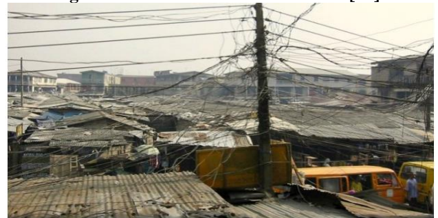
Figure 2: 0.415kV Distribution Network [29]
