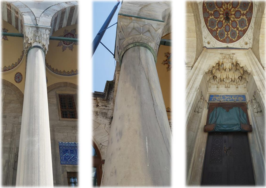
Figure 3: Example of muqarnas in the carrier system and door of Sokullu Mehmet Pasha Mosque.
