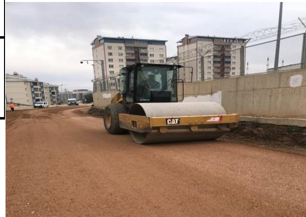
Figure 4. A subbase layer construction
