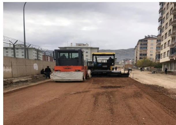
Figure 5. A base layer construction
