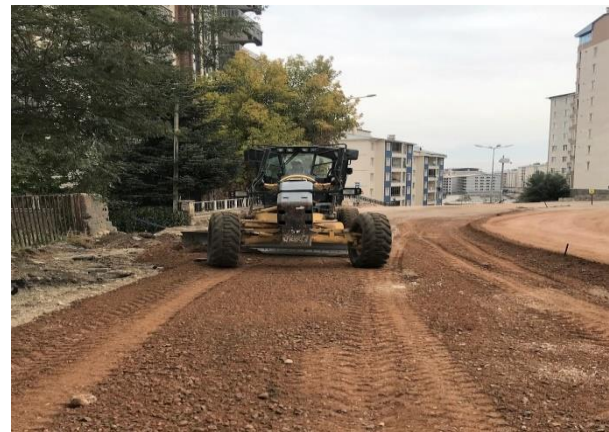
Figure 3. A subgrade construction
