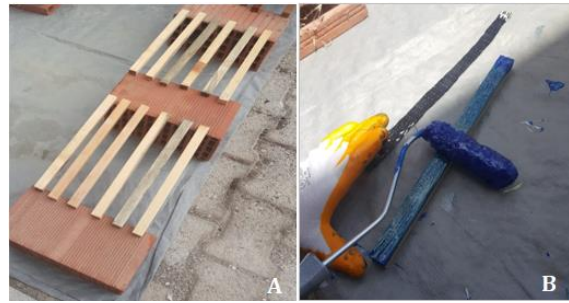
Figure 1 Image of the wrapping process with FRP polymers, A: Preparing the beams for wrapping after the priming process B: Wrapping the beams with FRP polymer fabric
