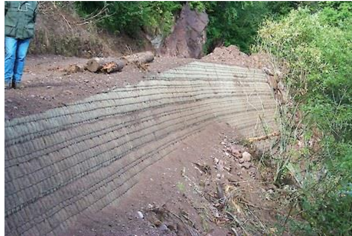
Figure 24. MSES Retaining wall.
