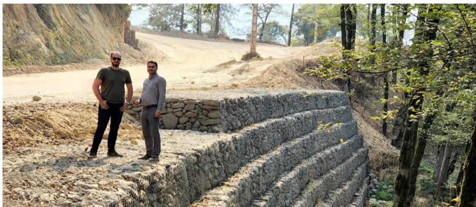
Figure 31. Km: 4+950 after construction and backfill
