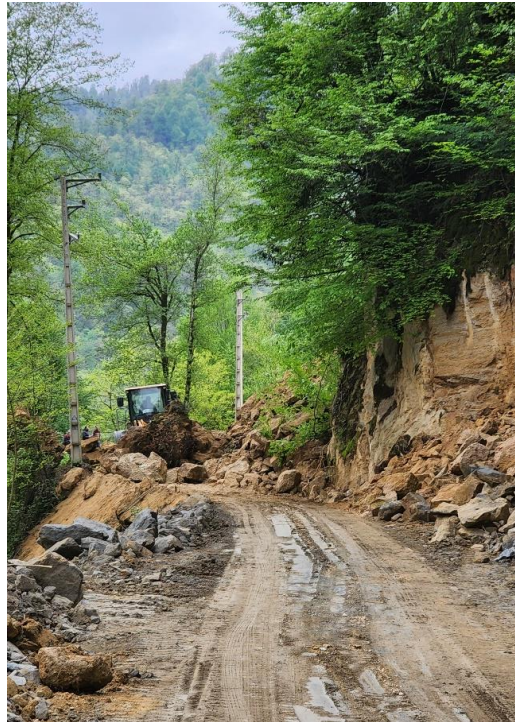
Figure 7. Goliran Road Widening
