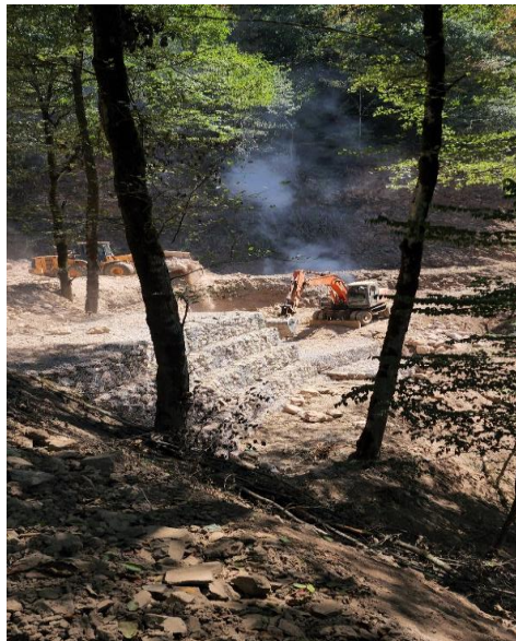
Figure 29. Retaining wall construction km 7+500
