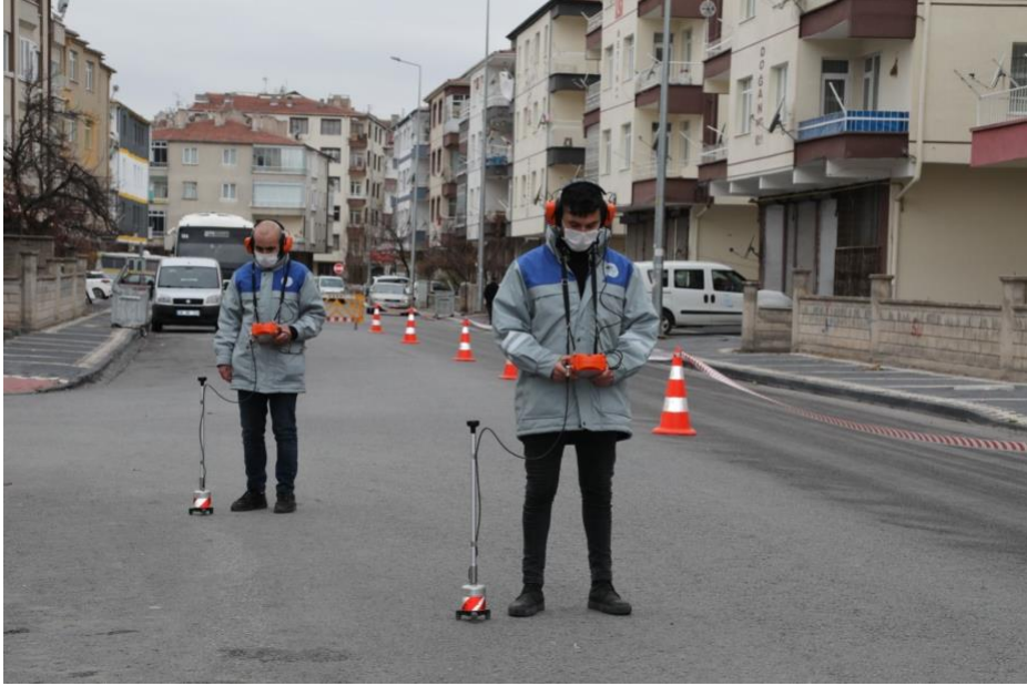
Figure 2: Sample Fault Detection Process with ground microphone
