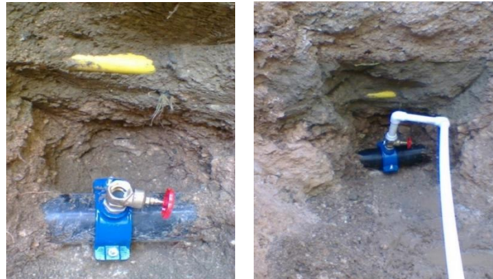
Figure 2. Service connection renewal in the field
