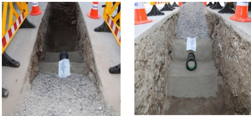
Figure 1. Network renewal in the field
