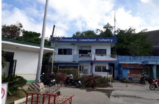
Photo 4: Jordan Wharf Ferry Terminal - Province of Guimaras (Photo Emin Atasoy)
