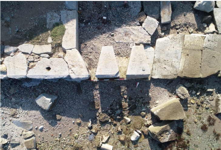
Fig. 9. Masonry Structure of the Northern Harbor Mole (Parion Archive).
