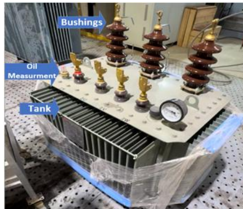
Figure 3. Transformer and its external components.
