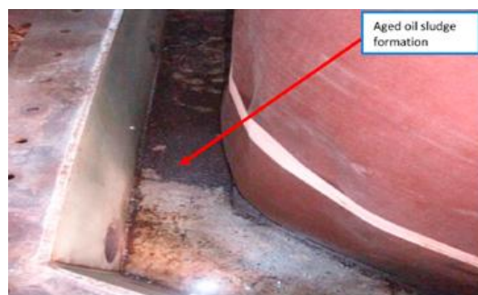
Figure 13. Older oil that has formed sludge [5]
